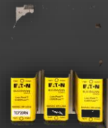
Main disconnect switch with high short circuit capacity. Optional cabinet door interlock.
